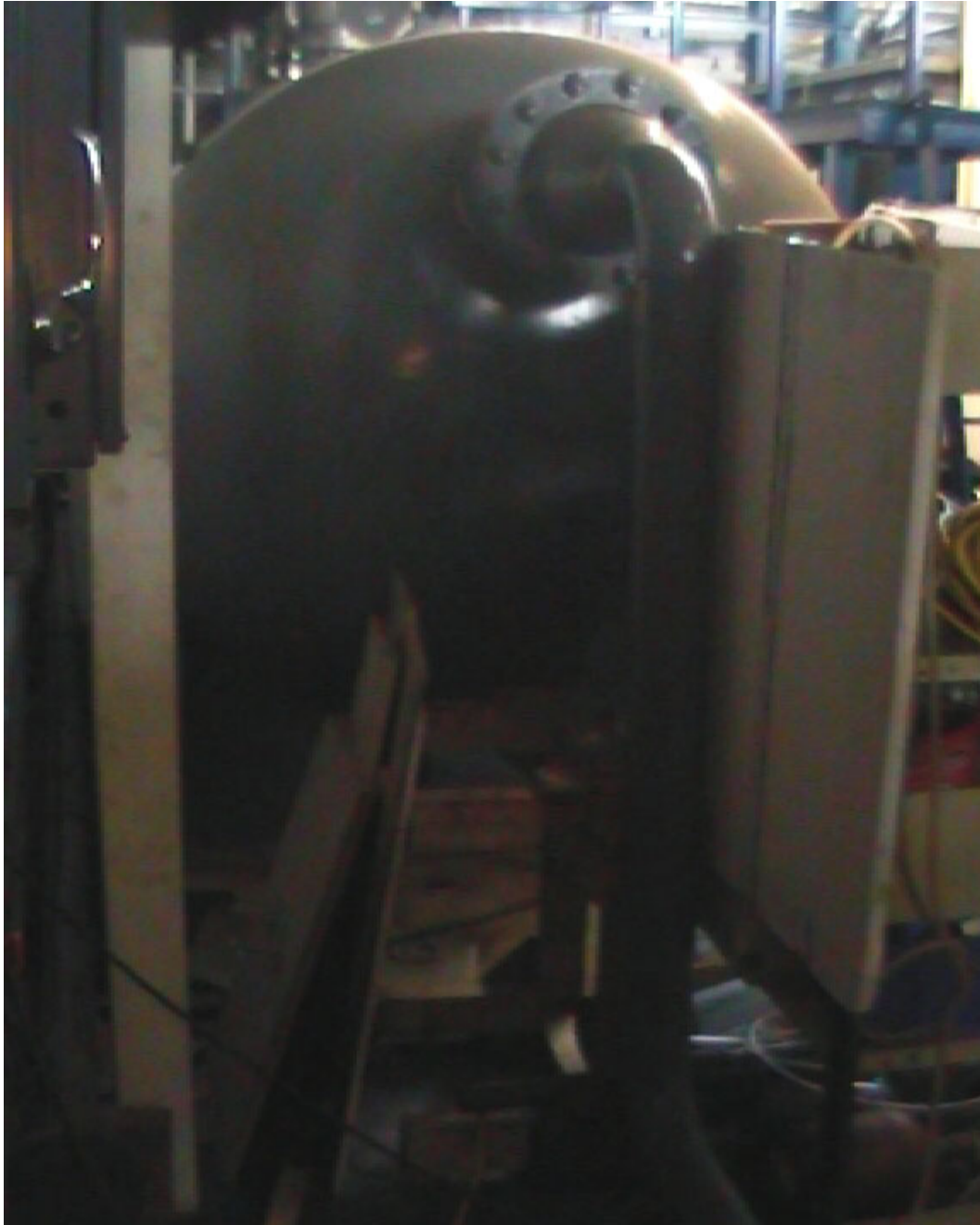
Figure 4.13: The slightly larger riser found at the end of the test section, where the pipeline enters the separator.
