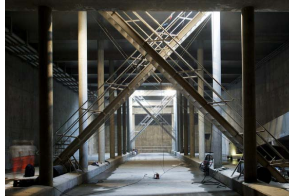
Basin at Skt. Annæ Plads in Copenhagen – Has a capacity of 8000 m 3
