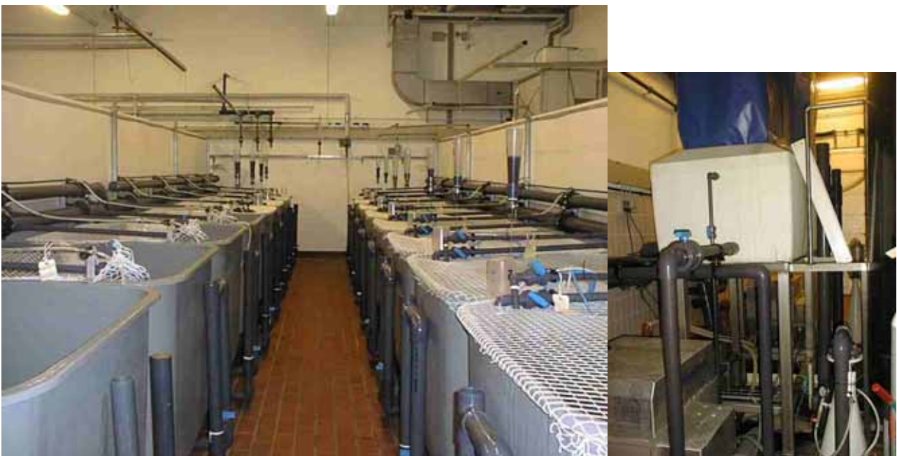
Figure 1. Experimental facility. The fish tanks were covered with net to prevent the fish from escaping/mixing between tanks. Above each tank a pendulum feeding machine was installed. The water treatment/purification was taken place behind the wall in the background (right picture), i.e. mechanical filter (bottom left), biofilter (black tank right side), trickling filter (with cover) and oxygenation cone (bottom right corner).
