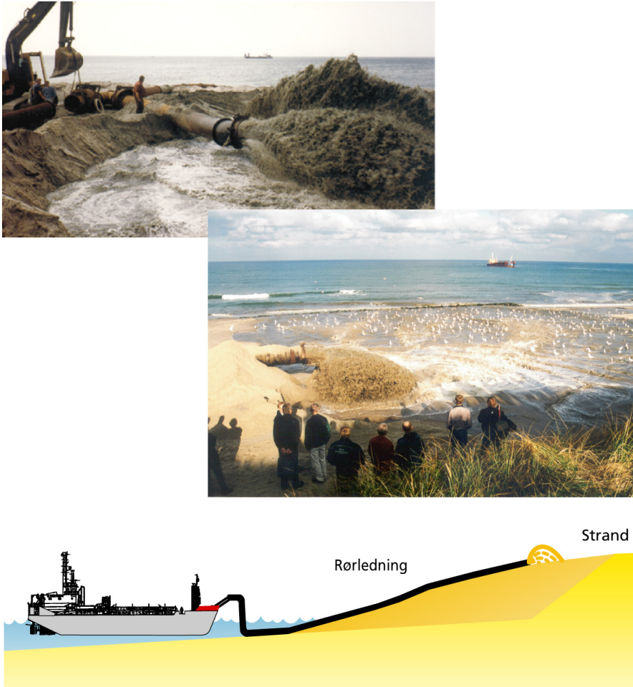
Figur 2.8. Princip strandfodring.
