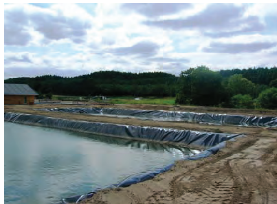
Figure 19. From the sludge cones, the sludge is transferred to sludge basins/tanks for settling of particulate matter. Left from Ejstrupholm Model Trout Farm (Photo Alfred Jokumsen) and right from Løjstrup Model Trout Farm. Photo: Lisbeth J. Plesner.
