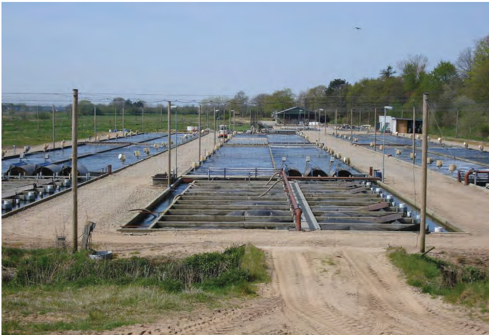
Figure 14. Kongeåens Model Trout Farm (type 3). The production units include three sections, each consisting of two concrete raceways with micro sieves (mesh size 74 \mu\text{m} ) in front of the biofilter sections (foreground). In the background to the left, the plant lagoons consisting of the former earthen ponds and the inlet and outlet channels are visible (Svendsen et al., 2008). Photo: Lars M. Svendsen.
