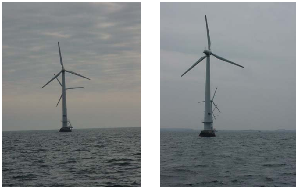
Figure 16. A perfect double wake (left) and quintuple wake (right). Despite the occurrence of these situations, it proved almost impossible to make measurements in these wake conditions due to the directional variability of the wind.
