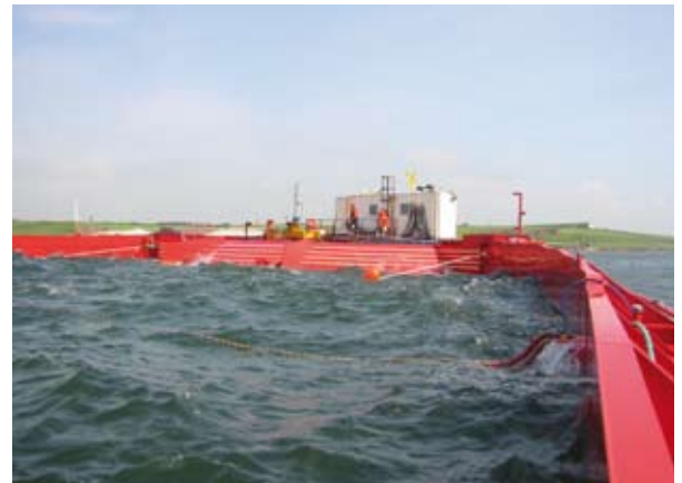
Figure 27: The Wave Dragon, a Danish wave power device.
