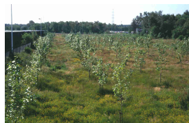
Figure 1. Installation of a phytoremediation barrier for the treatment of a BTEX-TCE plume. Phytoremediation will be done using hybrid poplar. Phytoremediation will be improved using modified endophytic bacteria.
