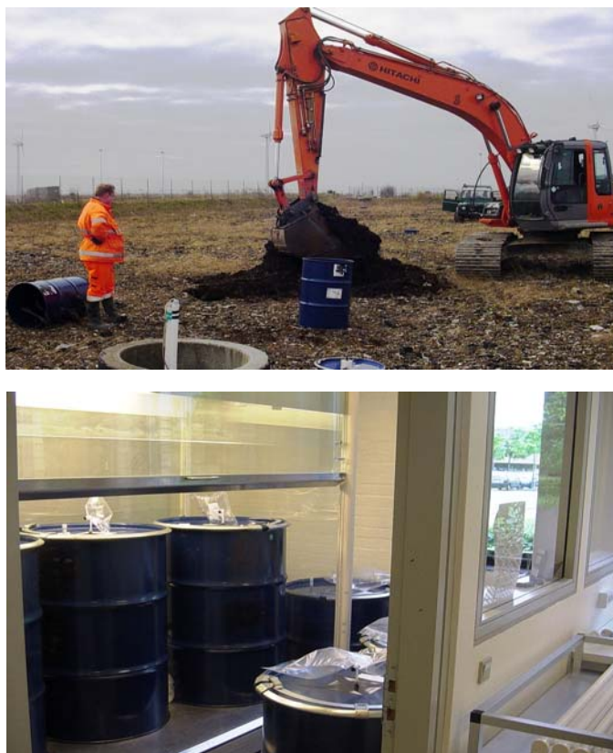
Figure 6.3. The top picture shows excavation of waste at cell 1.5.1 containing shredder waste AV Miljø. The bottom picture shows the experimental setup.
