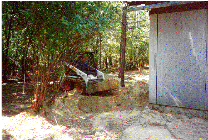
Plate 3.4. Application of clean sand at the corner of house number 1.
