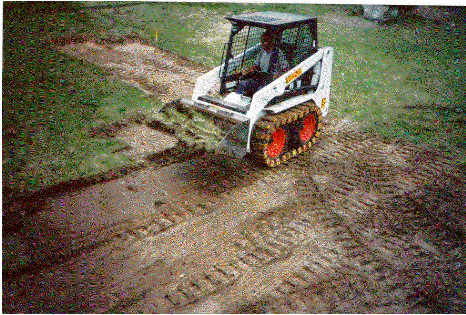
Plate 3.2. The first exercise with the Bobcat cleaning a grassed area close to the river bank.
