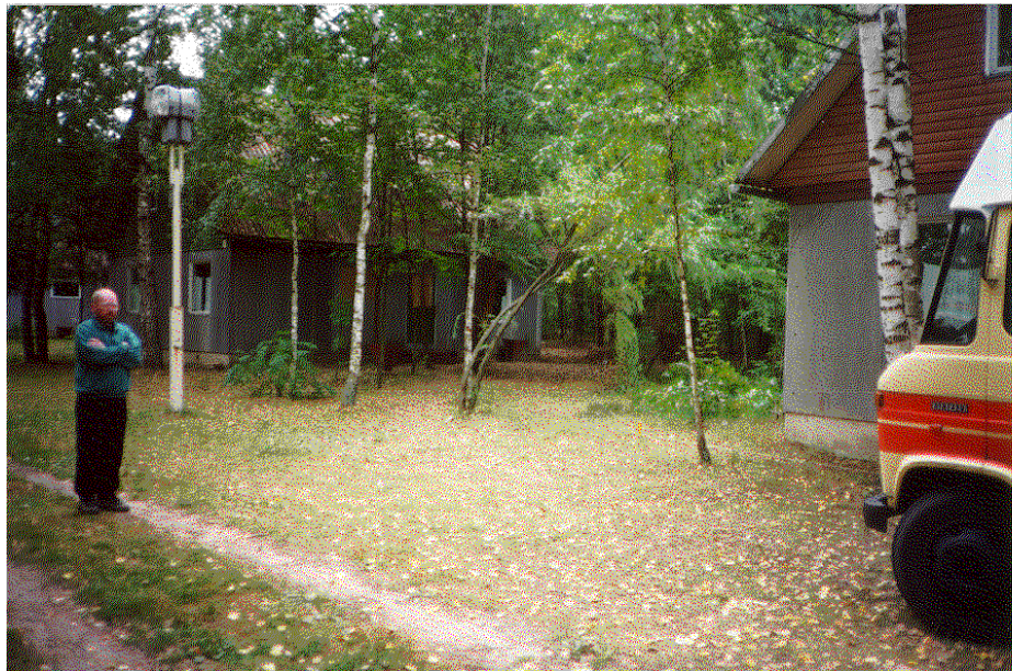
Plate 3.1. View of the houses before the decontamination. From the right to the left houses 1, 2 and 3 can be seen.
