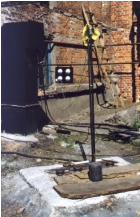
Figure 2.2 Measurement of the flow field and oxygen distribution in the duct. A similar method is used for sampling fly ash from the duct
