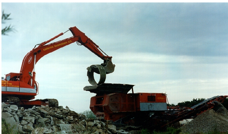
Figure 4.2. Crushing of concrete rings from the obsolete low-level storage facility 'Betonrørslageret'
