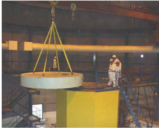
Figure 4.1. The 13-ton concrete shield is removed from the top of the reactor block on 25 May 2000. Below the concrete shield is a 10-cm lead shield.
