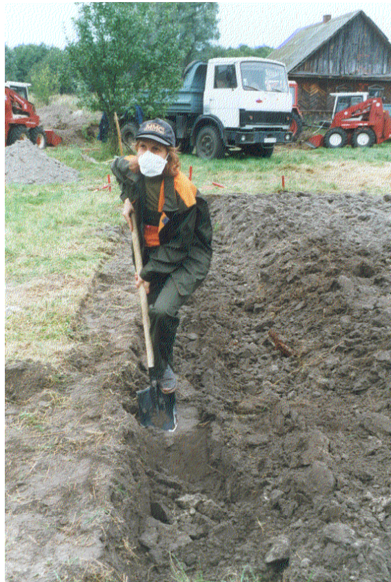
Figure 2.3. A representative of a Belarussian decontamination company gaining hands-on experience with the triple digging procedure in Savichi
