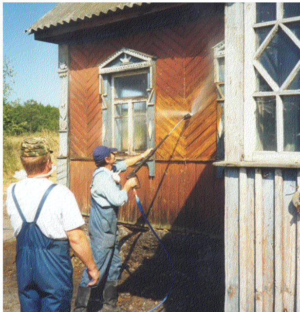
Figure 2.6. Local workers attempting to decontaminate a wooden wall in the strongly contaminated village of Savichi (Belarus) situated within the 30 km zone around the Chernobyl nuclear power plant. Decontamination of walls is generally only worthwhile in strongly contaminated areas. High-pressure water hosing requires that walls are waterproof. Safety precautions are often neglected if they are inconvenient for the work process.
