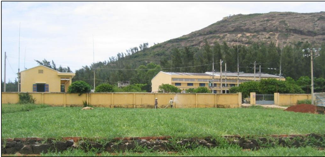
Figure 23: The diesel power plant at Ly Son. (Photo: RISO 2006)
