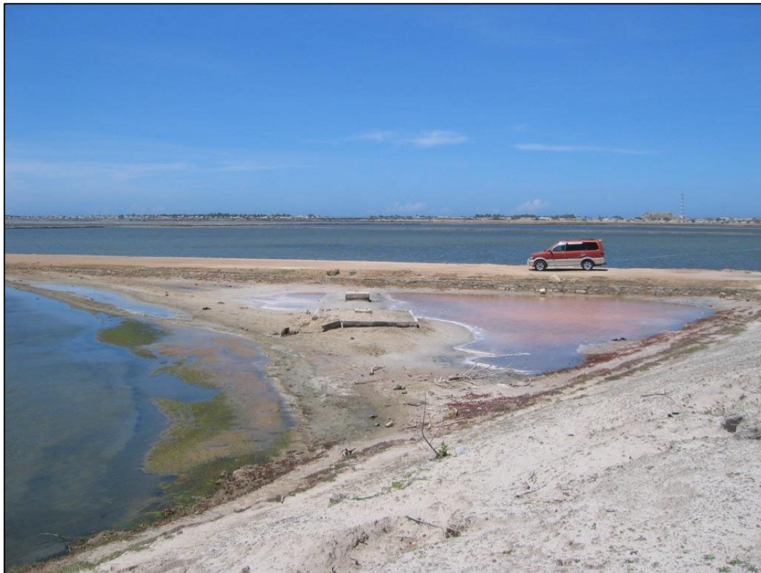
Figure 12: Site of the met-mast installed at Ca Na during June 1998 – June 1999, indicated by the foundation. (Photo: RISO)
