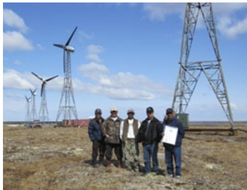
◀ Utility managers of the Chaninik Wind Group in front of wind turbines installed in Kongiganak
