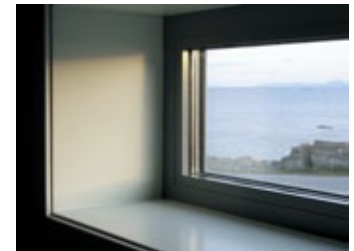
▲ Substantial wall insulation and energy efficient windows and lighting systems reduce the energy consumption of the centre
