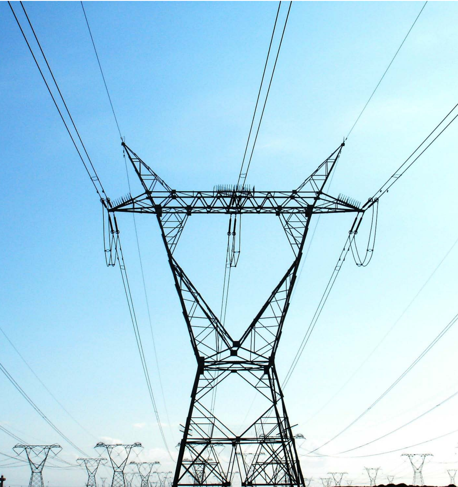
Transmission lines in South Africa Photo: URC internal archive
