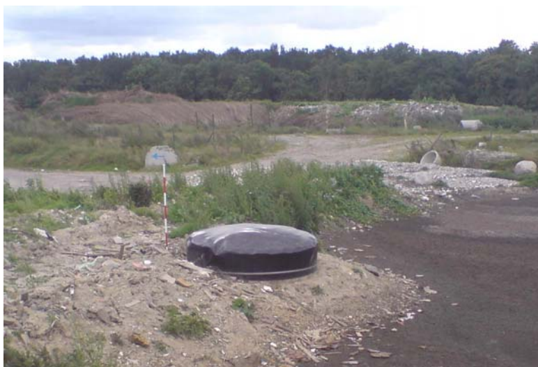
Figure 1.3. Cap on leachate well installed to prevent LFG emission. These flexible caps were seen to bulge out shortly after fitting them on the leachate wells.
