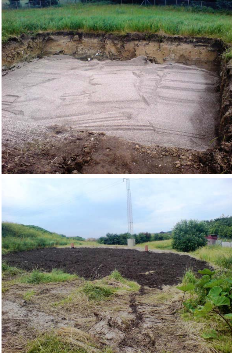
Figure 1.4. Biowindows during construction (top) and after construction (bottom).
