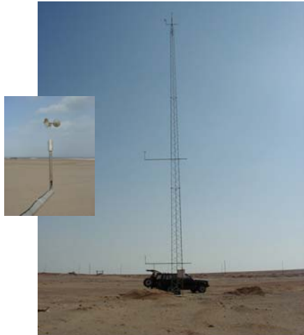
25-m lattice tower, concrete foundation
