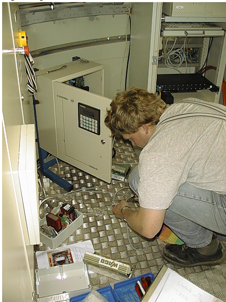
Figure 4: VIBRO-IC installation in the tower base of turbine 7.
