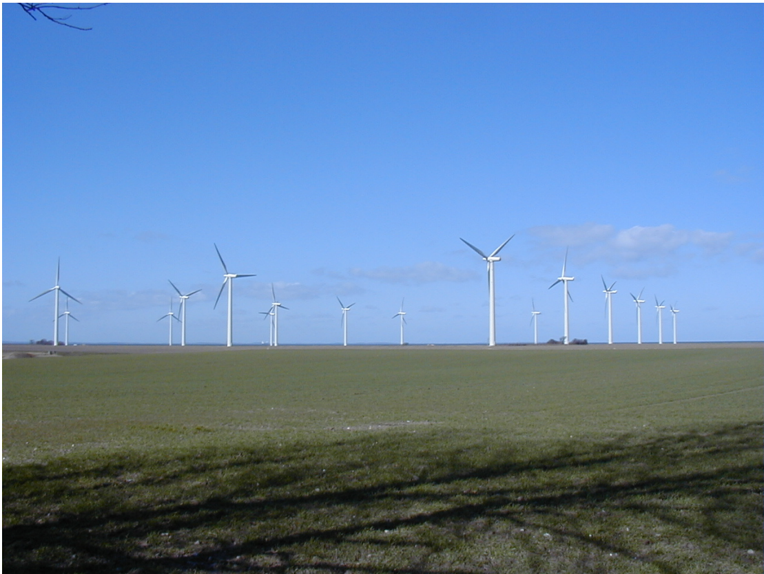
Figure 28: The wind farm at Nøjsomheds Odde on a particularly sunny day.
