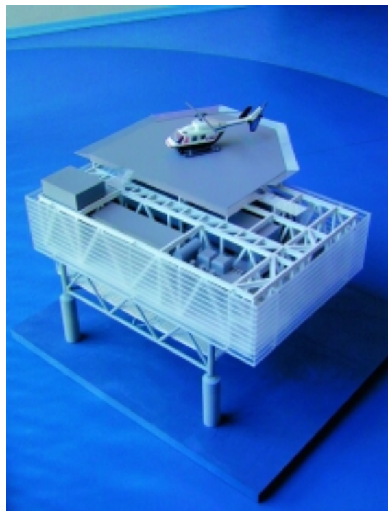
Figure 3. Offshore Transformer Substation Module.
