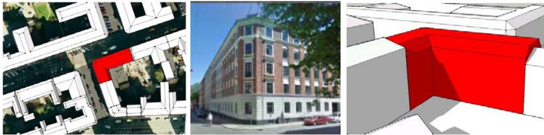
Fig. 13: Map showing the location of the case building in its context (to the left) and picture of the existing building showing the façades towards the street facing north and west
