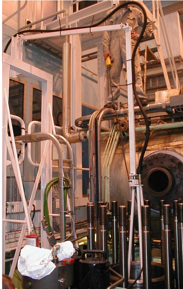
Figure 14.6: Overall view of tripod arrangement
