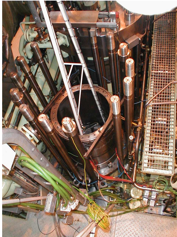
Figure 14.7: Closer view of tripod arrangement
