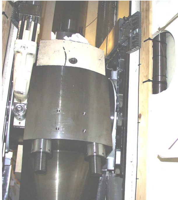
Figure 9.5: Measurement guide shoe installed in engine section
