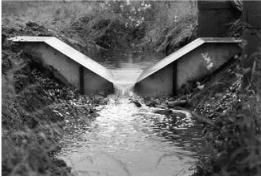
Figure A.2. Rounding of weir B carries the upstream energy level to its long crest, where hydrostatic conditions prevail until a submersion of 80 %, as monitored by the downstream stilling well. Braces, shelters, pebbles, and plastic membranes retard the erosion.
