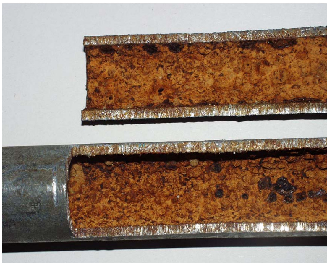
Figure 5. Encrustations in a typical drinking water pipe.
