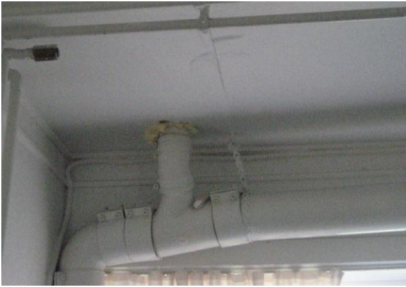
Fig. 30. Ceiling between two bathrooms, possibility of the humidity problems and cold floor
