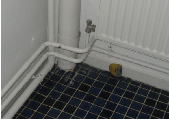
Fig. 32. Thermal bridge and cold floor along with corner in the bathroom in the basement floor
