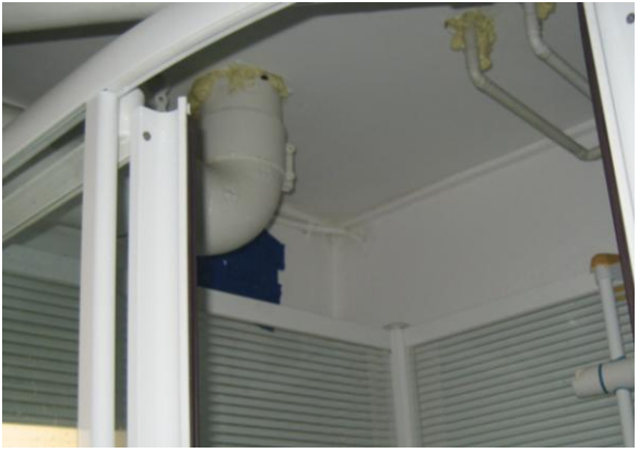
Fig. 31. Un tightness of the natural vent in the bathroom in the basement floor
