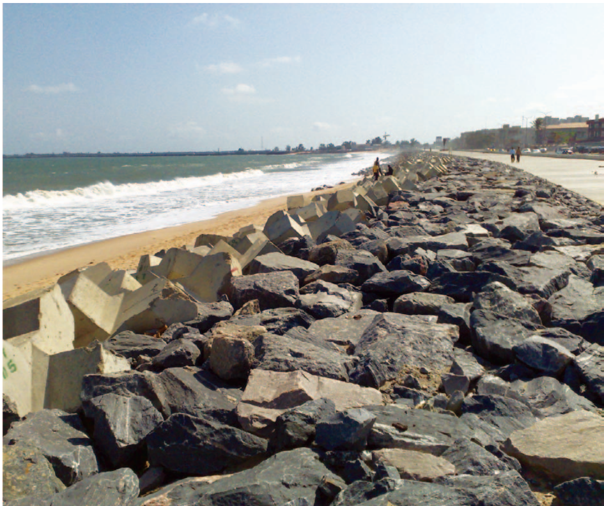
Figure 4.10: Bar Beach seawall, Victoria Island, Lagos, Nigeria
