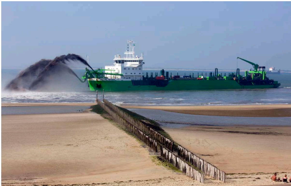
Figure 4.2: Rainbow method for transferring nourishment material ashore
