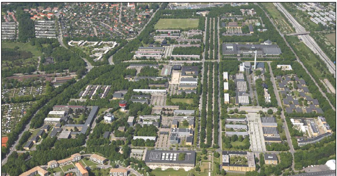
The Lundtofte Campus. The lab is close to the tall chimney.
