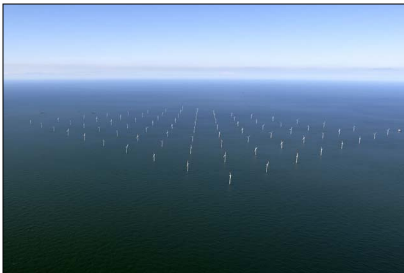
Figure 2.1. Horns Rev offshore wind farm. Courtesy of DONG energy.
