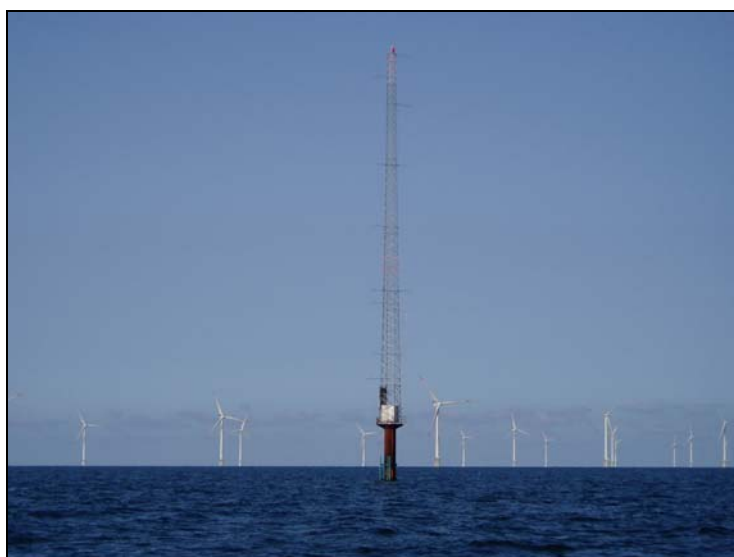
Figure 2.7. Photograph of M6. Courtesy of DONG energy.
