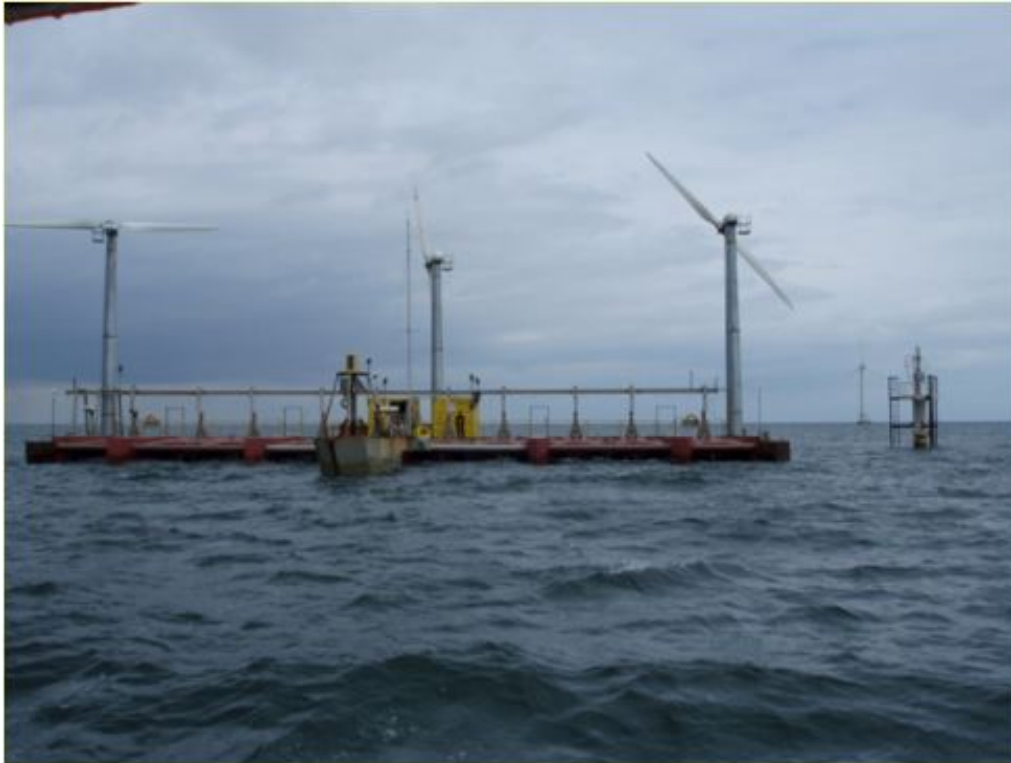
Figure 7: The Poseidon demonstration project is a floating power plant which harvests both wind and wave energy
