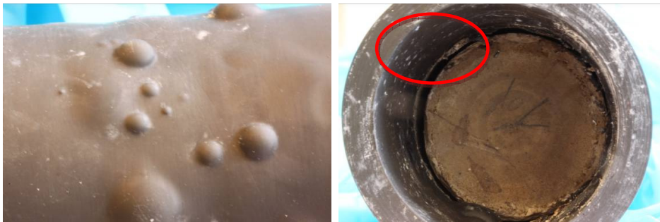
Figure 53 Broken rubber sleeve (core #7)
