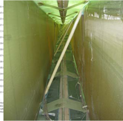
Figure 12. The assembled box girder with cap reinforcement in both upper and lower part and cross reinforcement between the corners.
