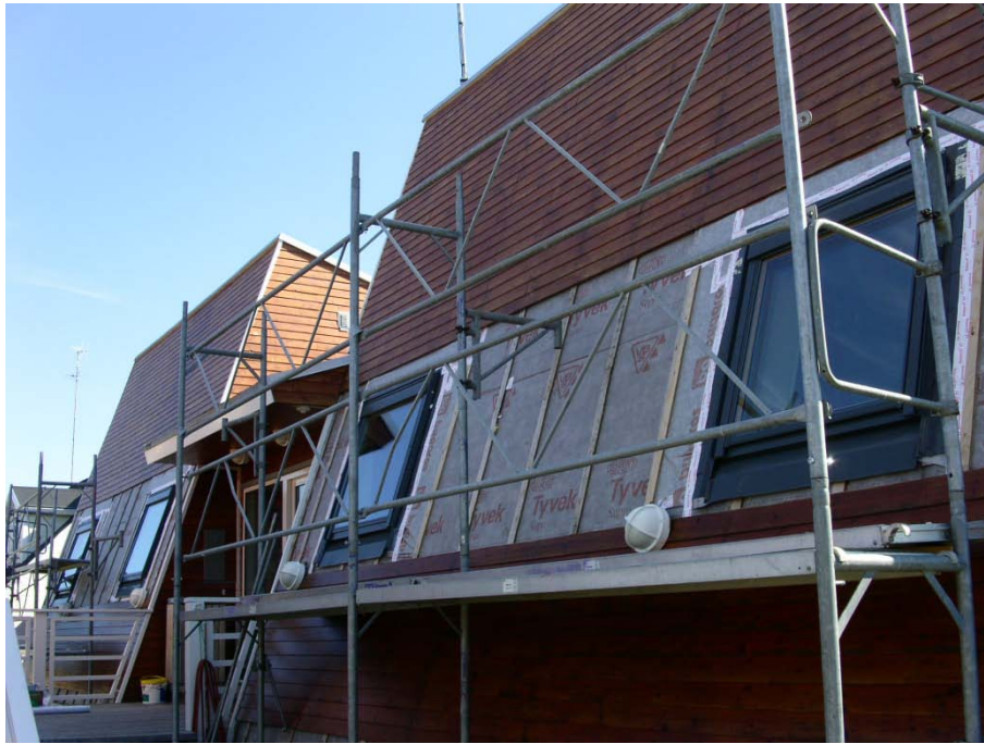
Improving the air tightness (summer 2010)
