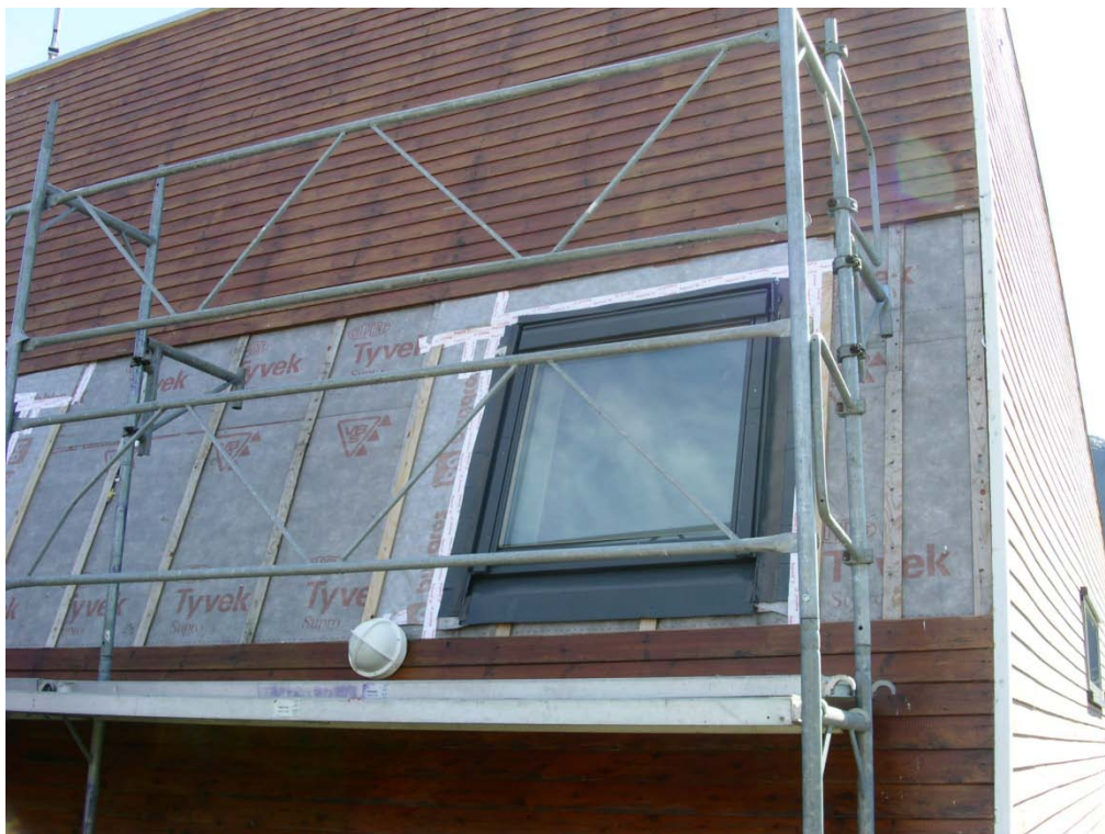
Improving the air tightness (summer 2010)
