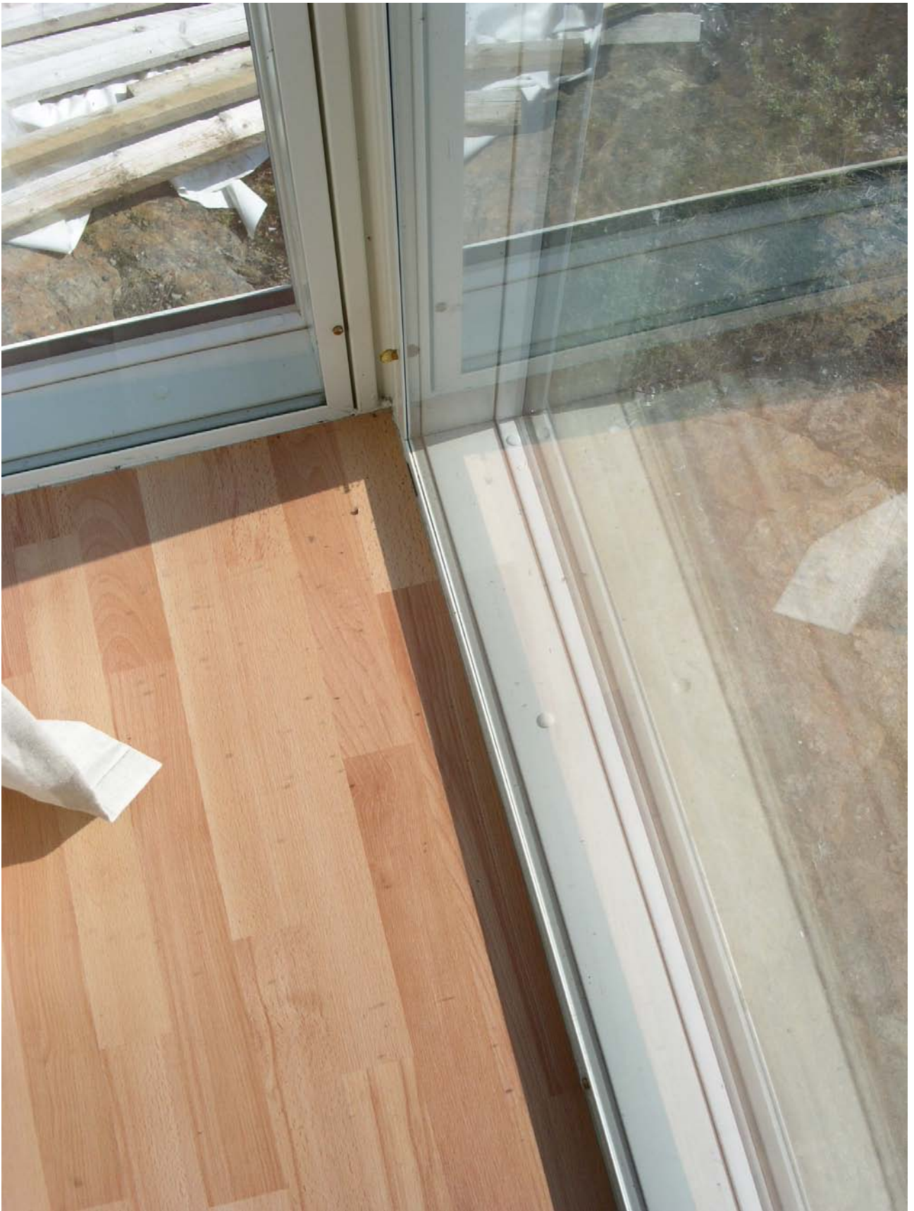
Sealed holes in the window frames.
