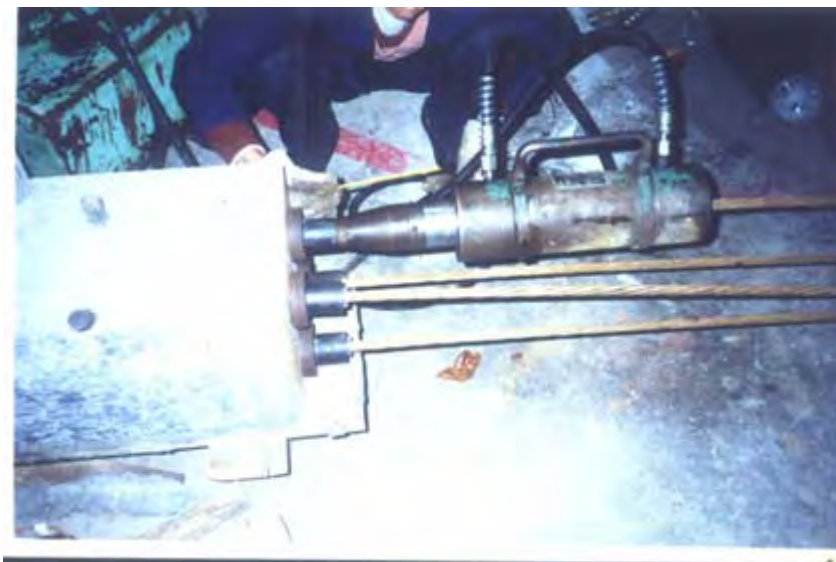
Fig.2.3 The process of tensioning and grouting
