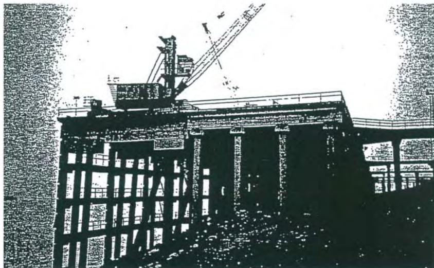
Fig.1.3 Wharf supported on piles of Wuhan Port
