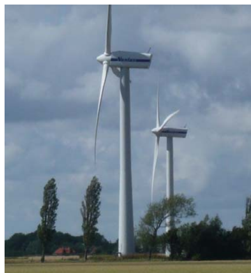
Figure 2 Often seen in the landscape: wind turbines that deviate significantly in yawing direction
