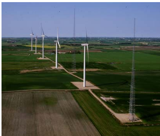
Figure 1 The row of wind turbines at Høvsøre with the 116.5m meteorological tower in the foreground and the 160m beacon mast between the first and second wind turbine. The picture is taken from a low flying aircraft to the south-west of the mast.
