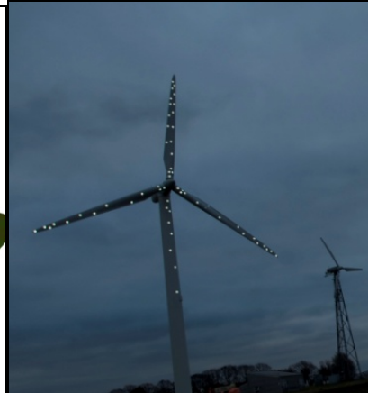
Figure 5 The effect of flash on the reflective markers. Wind turbine at campus, Dec 2007.
