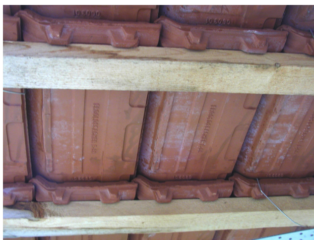
Figure 5.24: After exposure to natural weathering the backside of tiles with Lotus Effect have a white covering.
