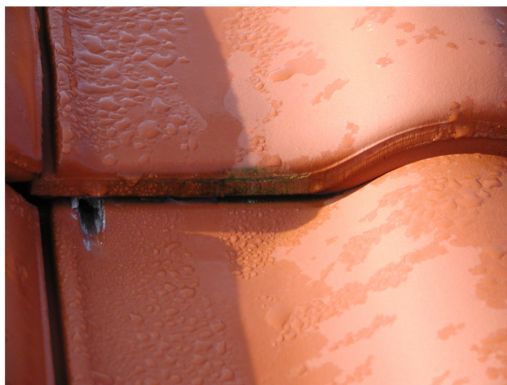
Figure 5.2: After 1 year a greenish layer became visible at the edges of north facing ordinary tiles (morning picture).
