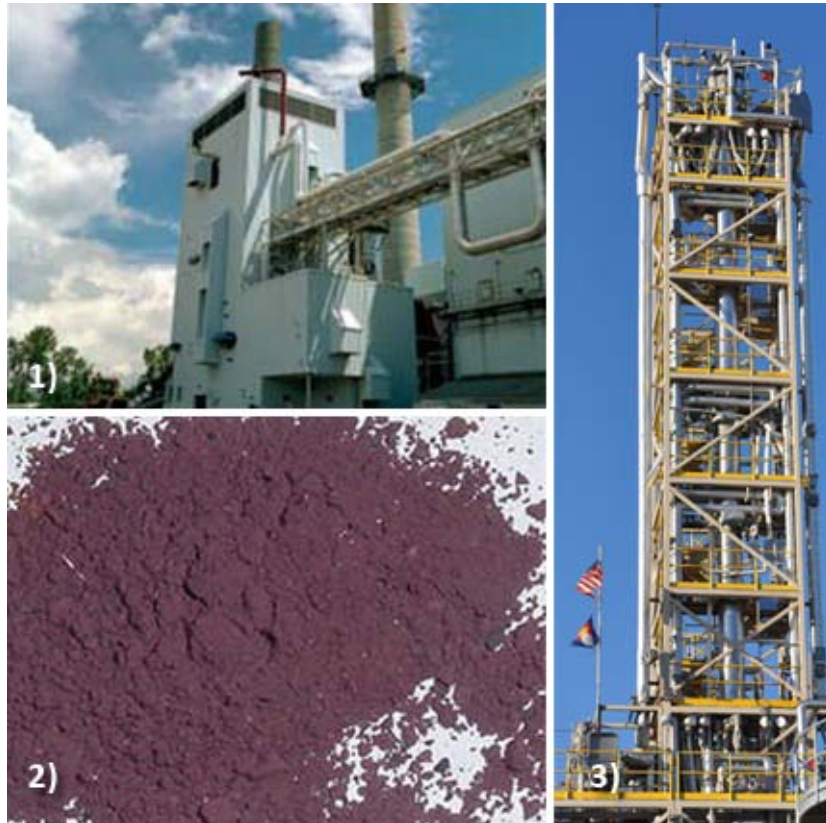
Figure 3-11: Picture 1) Vermont Gasifier of the SilvaGas type. Picture 2) Rentech process iron-oxide catalyst. Picture 3) Rentech Reactor for methanation or other fuel synthesis (Rentech, 2009)
