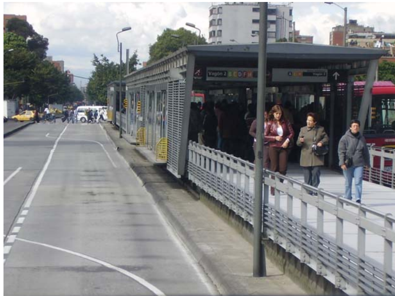
Figure 3: Transmilenio Bus Station Picture: Andrés Valderrama
