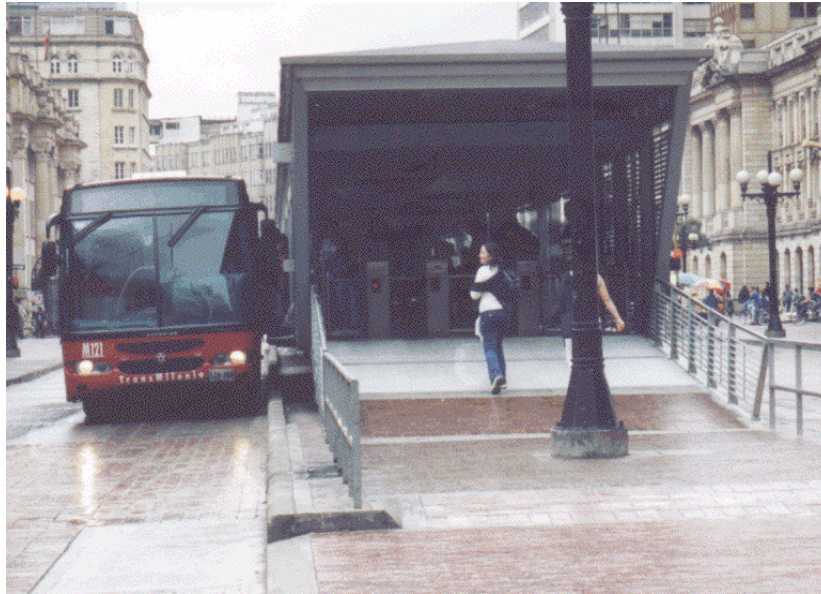
Figure 3. Picture showing the ramp to the station and the levelled access between the station and the bus. Picture taken from Rickert (2008)
