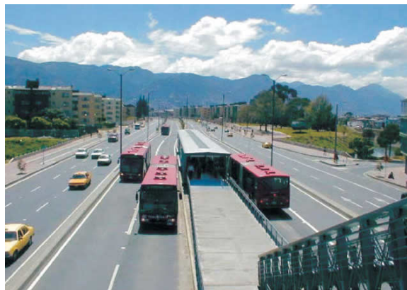
Figure 3: Picture of the system to illustrate how the bus traffic is separated from the private car, the public taxi, and the service traffic. Stations are in the middle of the road and the access is provide by pedestrian bridges. Picture retrieved from Transmilenio S. A. web page http://www.transmilenio.gov.co/transmilenio/frameset_gneral.htm the 27th of April of 2006.
