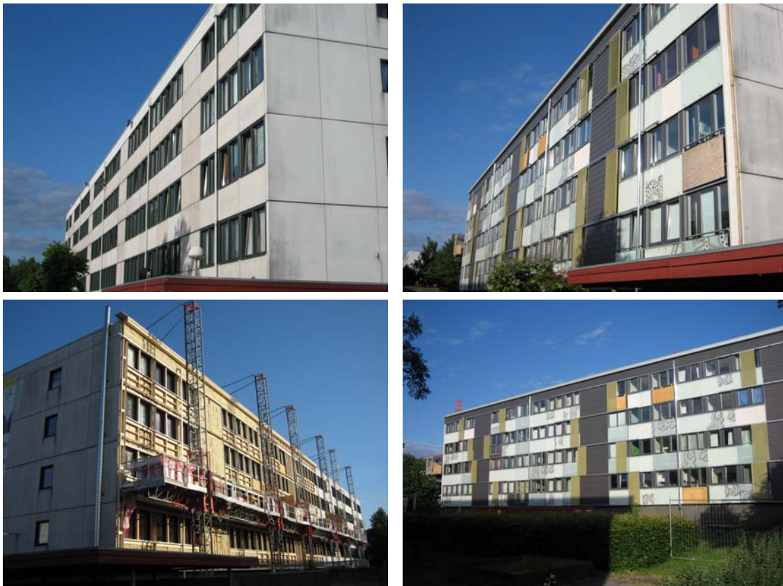
Figure 40. Garden side façades on Remisevænget Øst before, under, and after works (Gottlieb).
