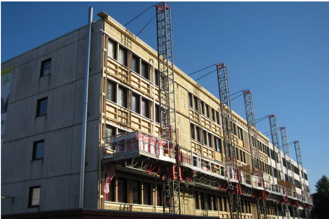
Figure 53. Work cycles, flow and stages of completion.
