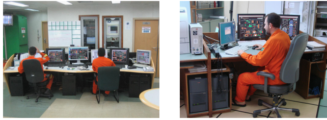
Figure 4: CPUs positioned under the counters, limiting the space for operators' legs
