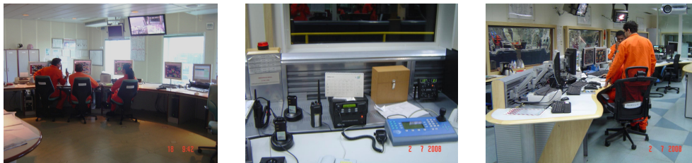
Figure 3: Consoles fitting up to two people, with space for placing the equipment over the consoles and with articulated supports for the LCD monitors
