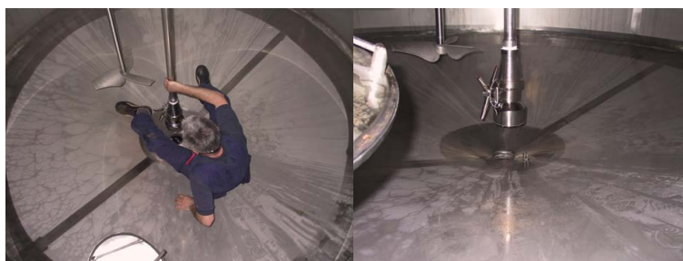
Figure A.2. The inside of the tank used for dissolving NaCl in sugar syrup. Both the impeller and the IM20 rotary jet head are seen.
