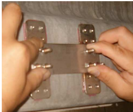
Figure H.6: Installing the mounts on a bridge-girder.
