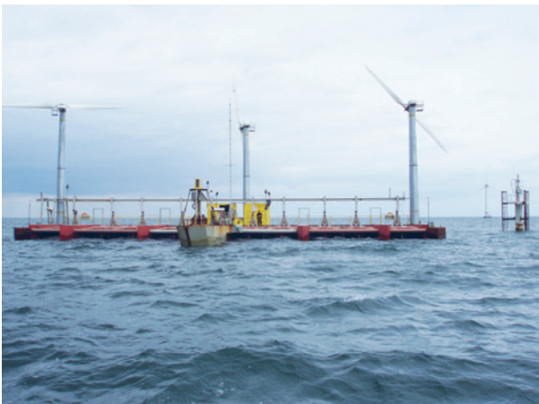
Figure 24: The Poseidon demonstration project is a floating power plant which harvests both wind and wave energy
