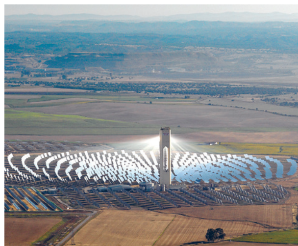
Figure 16: Planta Solar 10 or PS10 solar power tower in Sanlúcar la Mayor near Seville, Spain. 624 heliostats of 120 square metres focus the sun rays on the top of the 115-metre-high tower, where the receiver generates pressurised steam to run a conventional power cycle with 11 MW capacity.
