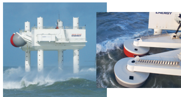
Figure 27: The two-float Wave Star prototype at Roshage, Hanstholm, Denmark
