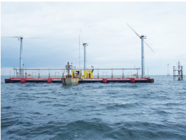
Figure 24: The Poseidon demonstration project is a floating power plant which harvests both wind and wave energy
