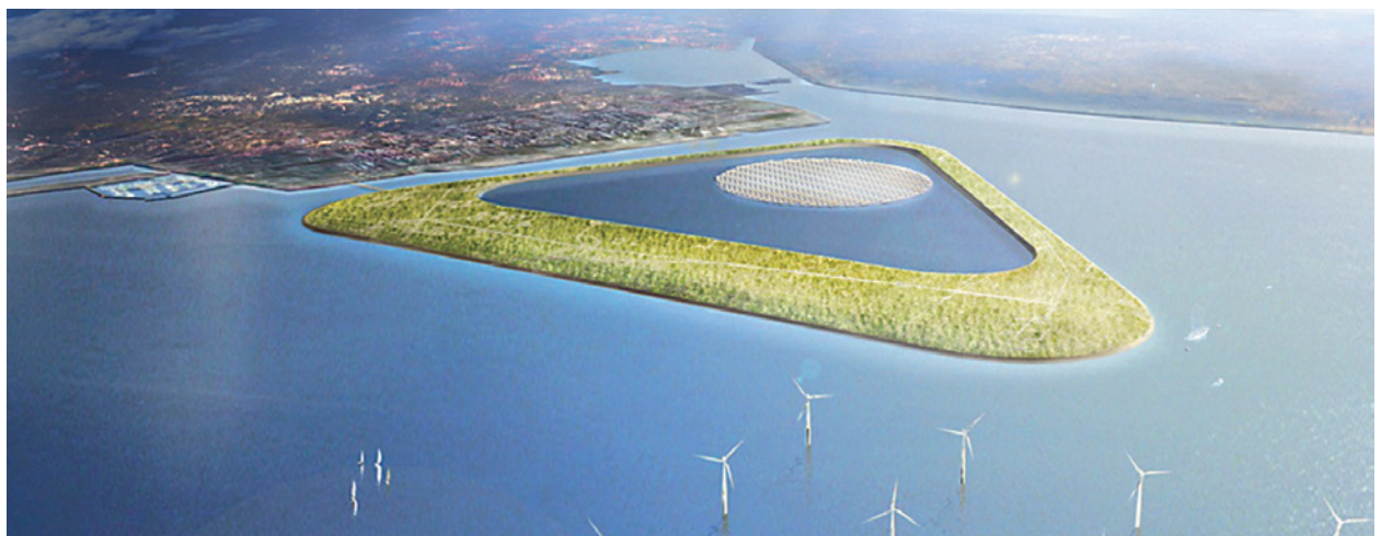
Figure 36: Artist's impression of an energy island. At the centre is a deep reservoir from which water is pumped out when electricity is plentiful. The electricity is later regenerated by turbines through which water flows back into the reservoir. The concept could be expanded with solar cells (circle in the middle) and algae production (source: Gottlieb Paludan Architects)
