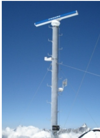
Figure 5.4 LAWR installation at the Klein Matterhorn, Switzerland. The LAWR is used for research by ETH Zürich, Institute of Environmental Engineering (IfU)
