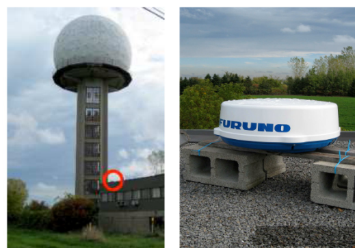
Figure 1 LAWR installed on the roof of the J.S. Marshall Radar Observatory next to the McGill S-band radar. Close up of the LAWR antenna unit on the right. The red circle shows the location of the LAWR.
