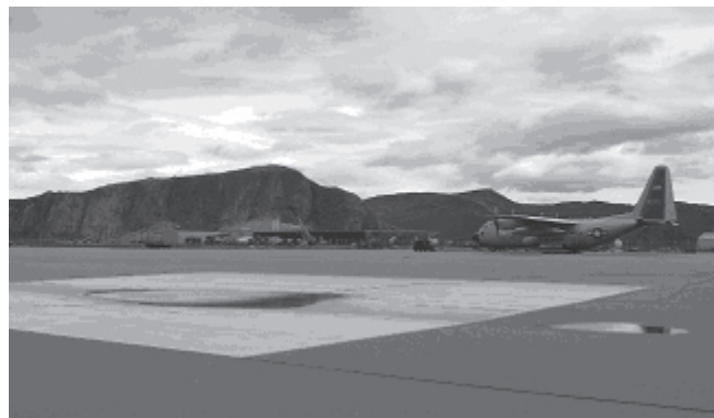
Figure 3A. White painted asphalt surface on the southern parking area of Kangerlussuaq Airport.
