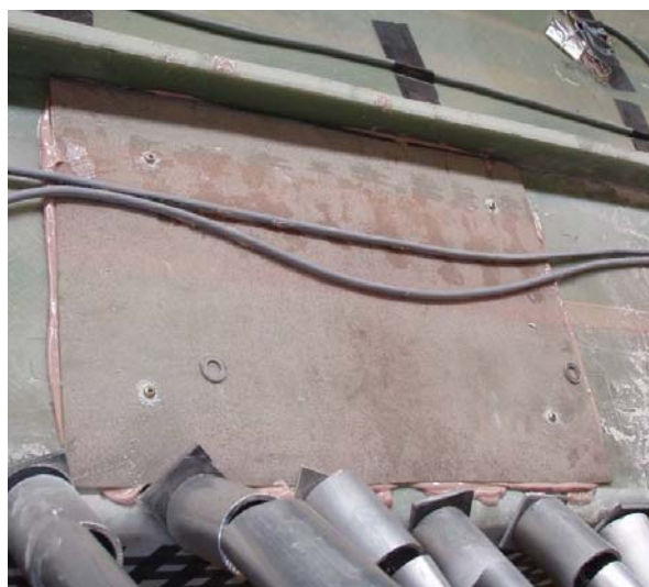
Figure 23. Repair damage on the shear web in the area 10.7m - 11.5m
