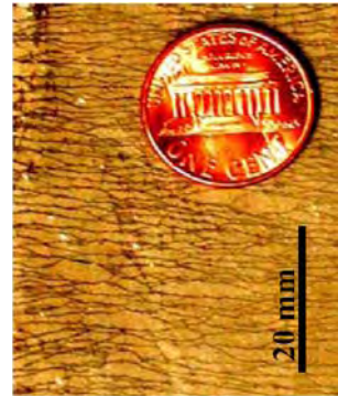
(b) Multiple cracks in ECC-specimen (Li &amp; Wang 2005).
